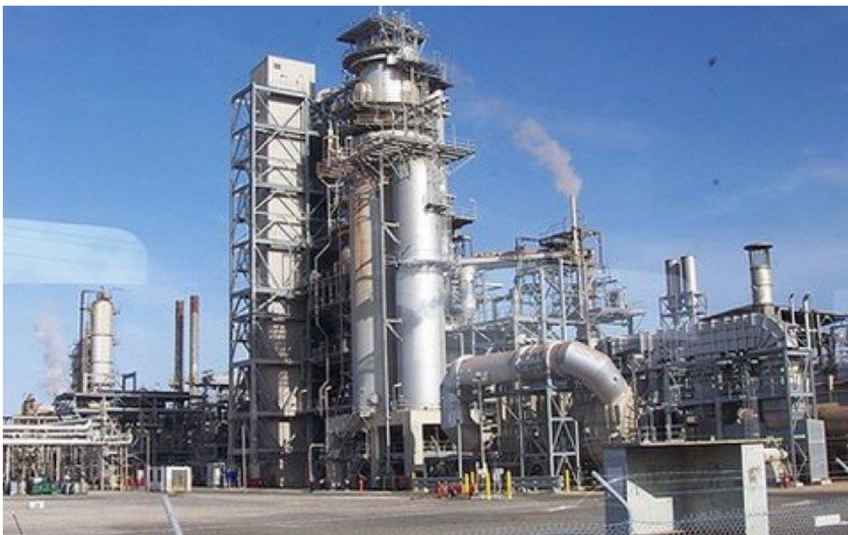
Figure 1: The Commissioned Gas Processing Plant at Atuabo
