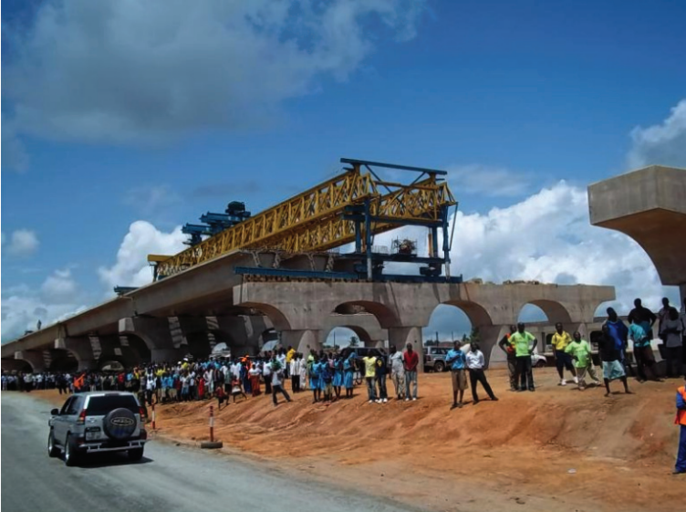
Work progressing on the Tetteh Quarshie – Madina Road
