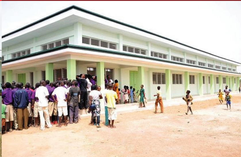
Newly built dining hall for Zebilla SHS
