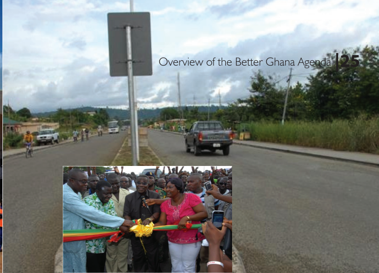
Commissioning of Koforidua Bypass
